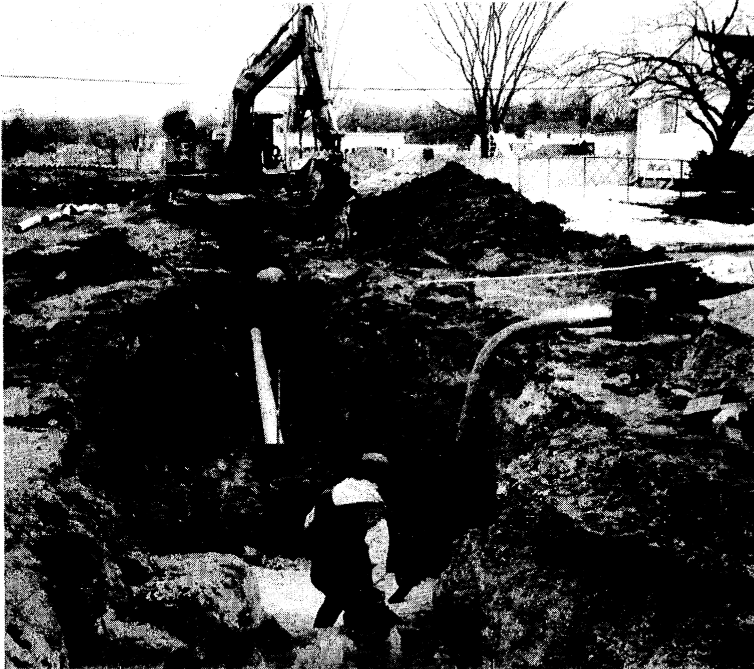
CARL ST. is finally going to be more than just a curb cut on Arthur St. The road was dug up last week as part of the Bridgetown Condominium project. It will provide a secondary access to the project. The main entrance will be off the Taylor St. extension on the opposite side of the project.
